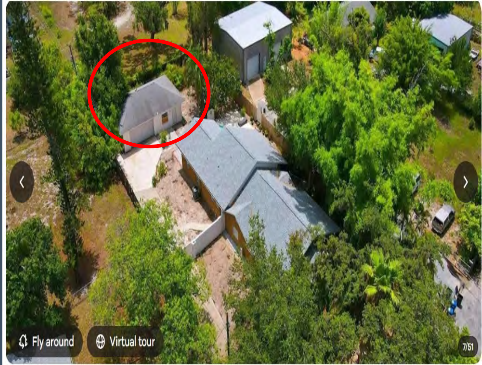
Aerial view of the garage prior to enclosure.
