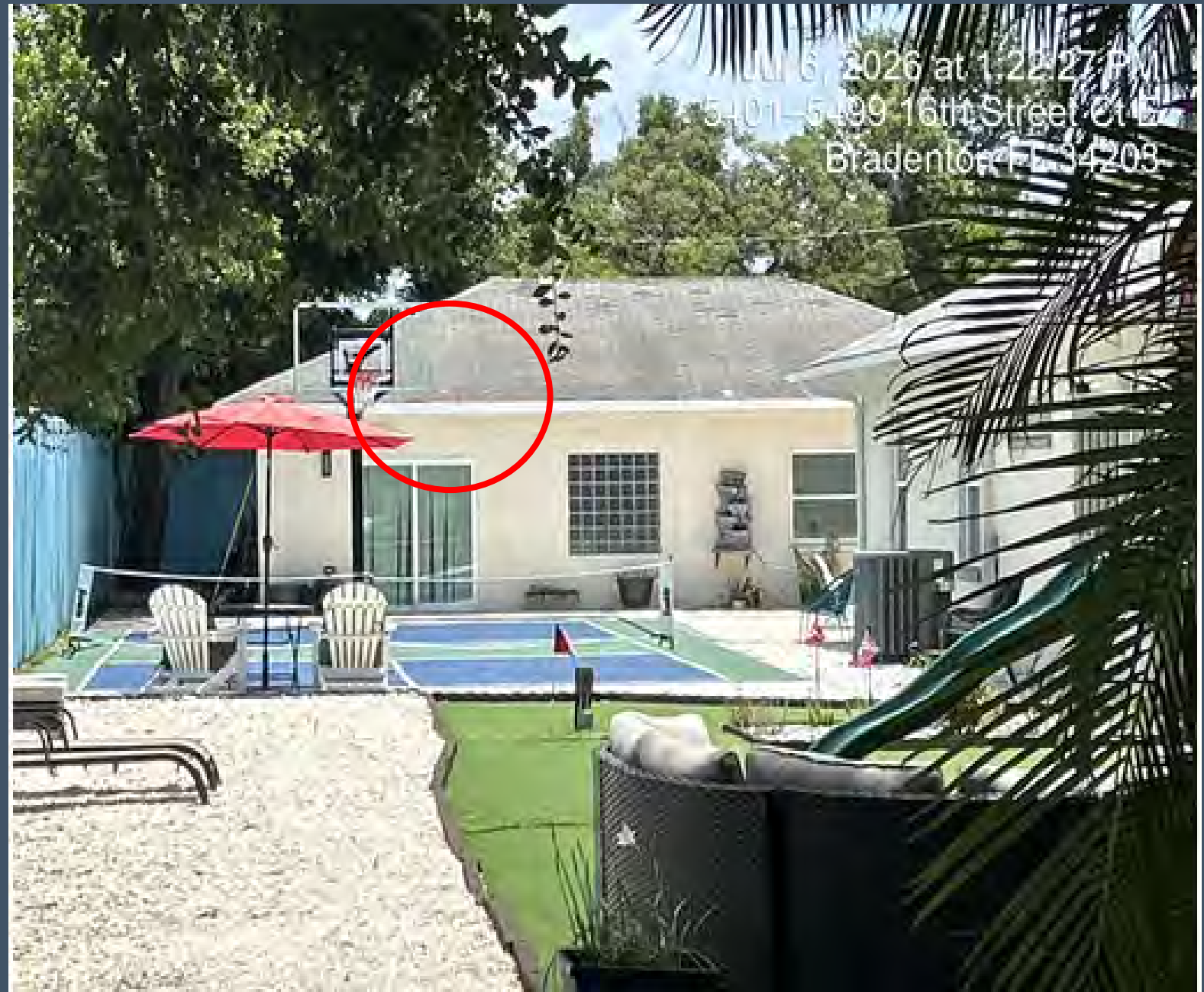
View of the now enclosed garage.
